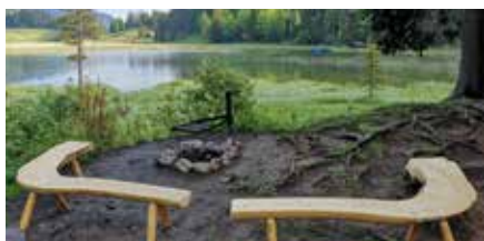
Construction and renovation of numerous leisure and barbecue areas.
