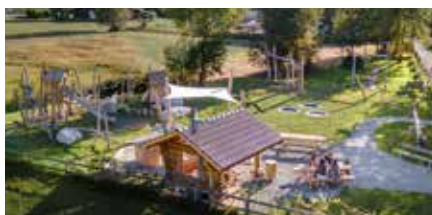
Construction of a new playground in Schönried.
